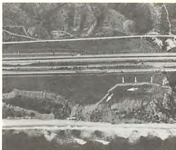
Figure 3. "After" photo, taken in February 1980. Landslide, measuring 700 feet long by 300-320 feet wide, occurred during the winter of 1978. Small arrows point to head scarp, and large arrows indicate direction of debris movement toward beach. (Photo: SIO Photo Lab.)
