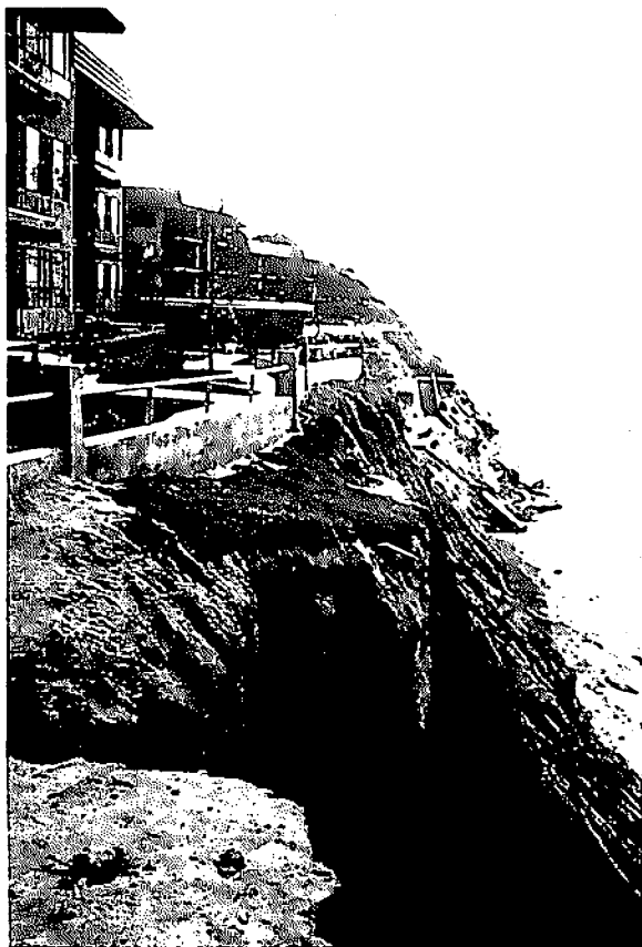
Fig. 1. Severe gulying of the sea cliff due to uncontrolled water runoff
