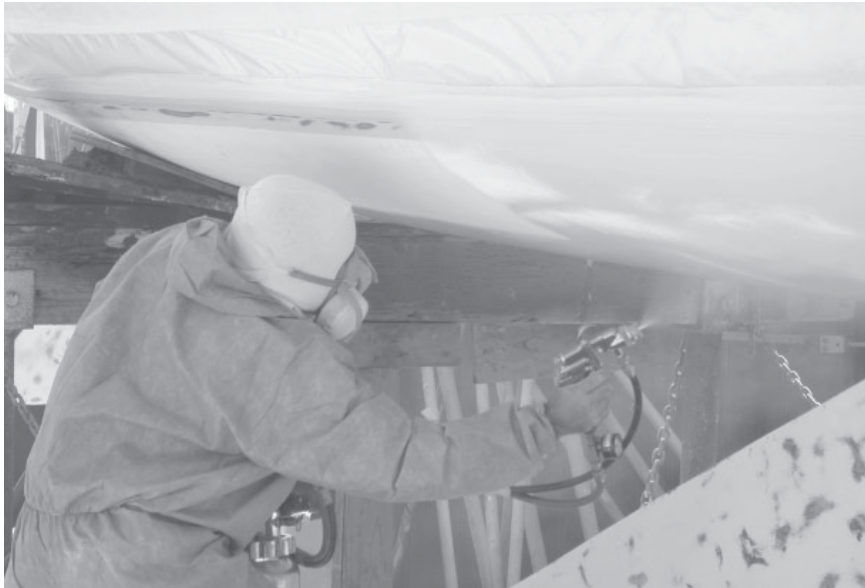
Nontoxic bottom paint being applied to boat hull. Photo: Jamie Miller, California Sea Grant Extension Program
