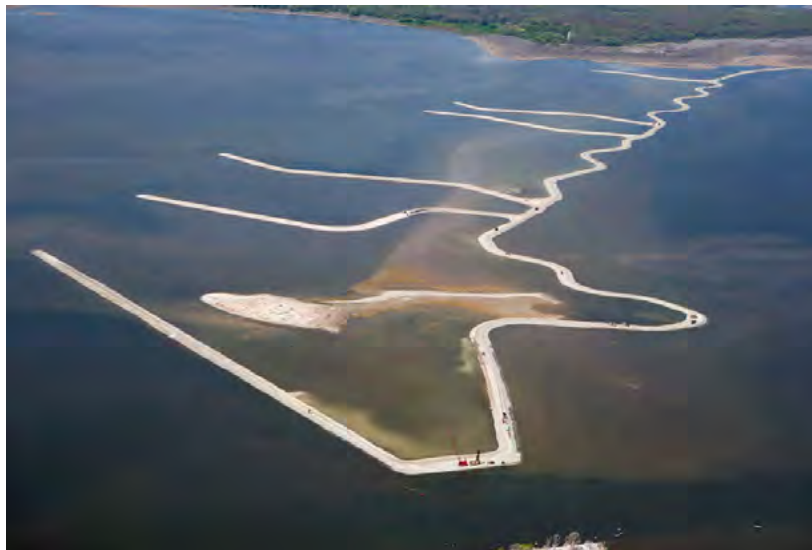
Figure 91: Cat Island spine construction, May 2013.
