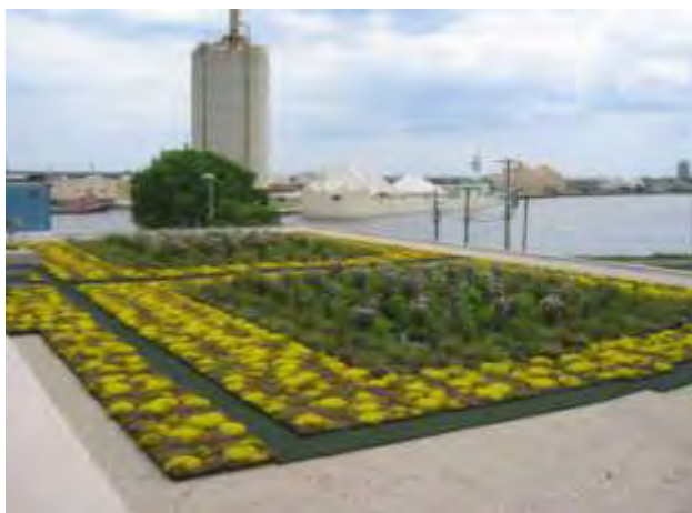
Figure ES-5. Green roof at the GLWI; a demonstration project to highlight strategies for mitigating stormwater runoff.
