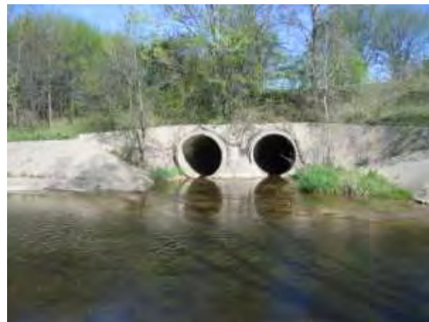
Figure 2: Example of Stormwater Outfalls.
