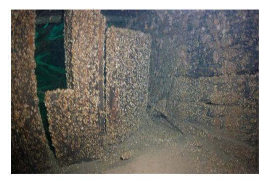
Figure 15. Port side bulkhead and door between the forecastle and cargo hold, looking aft.
