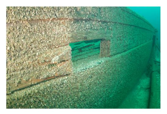
Figure 17. Forwardmost lumber port on the port side with two extant hinges. The freeing port is visible along the bottom of the bulwark, as well as the two thicknesses of bulwark planks.
