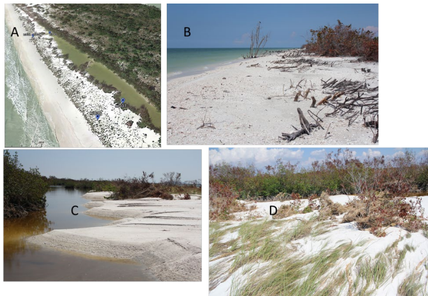
Figure 4. Beach erosion and overwash observed on Keewaydin Island after Hurricane Irma.
