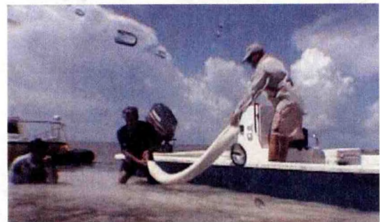
Figure 7. A shallow draft vessel was maneuvered close to the propeller scar and the sediment tubes were lowered into place.
