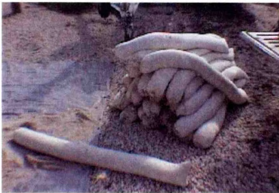
Figure 2. Filled sediment tubes ready to be deployed.
