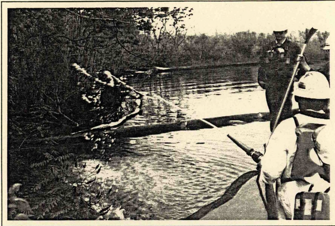
FIGURE 3. The spray nozzle and rate used to apply the Elastol to the oil.
