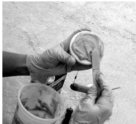
Figure 2: Apply a thick coat of the mixed epoxy onto the flat, bottom part of the white base-plate.
