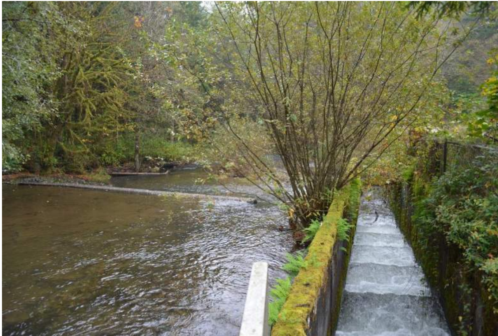
Figure 1. Downstream view of fish ladder and weir with pool behind weir. (Biological Assessment for Abernathy FTC Intake Upgrades, Prepared by Linda Mark, KPFF Project #1900372)
