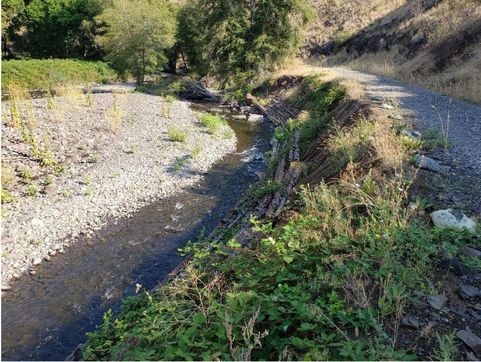
Figure 1. Photograph looking downstream at the side channel eroding stream bank and access road to the Chief Joseph Wildlife Area. The side channel rejoins the main channel at the end of the gravel bar.
