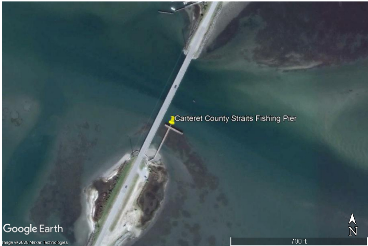
Figure 3. Carteret County Straits Fishing Pier and surrounding area (©2020 Google Earth)
