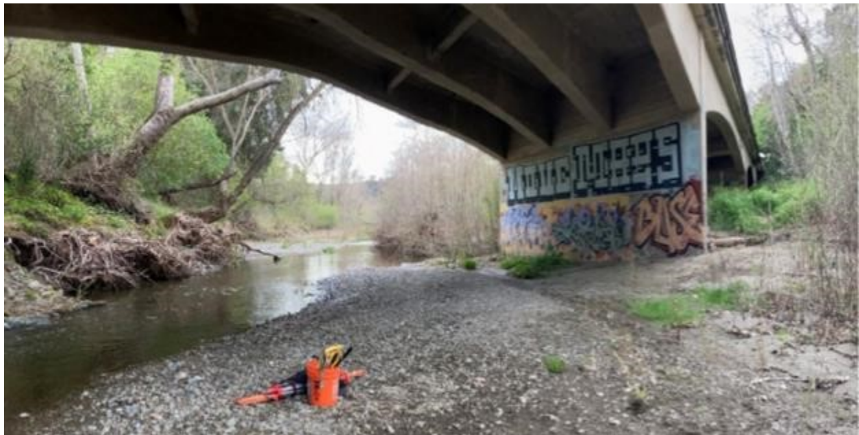
Photo 1. Existing bridge looking downstream (southeast). Source: Caltrans BA (2021).
