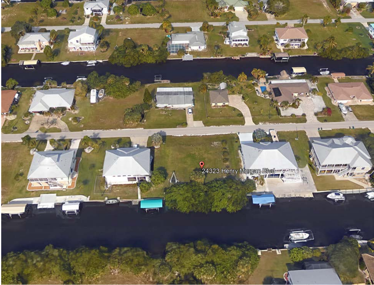
Figure 1. The McClung Seawall project site at 24223 Henry Morgan Boulevard, Punta Gorda, Charlotte County, Florida (©2018 Google).
