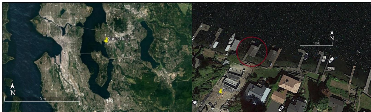
Figure 1. Google Earth photographs of the project site. The left image is a view of the project site on the eastern shore of Lake Washington in relation to Seattle to the west. The right image is zoomed in to show details of the project site, with the dock encircled in red.
