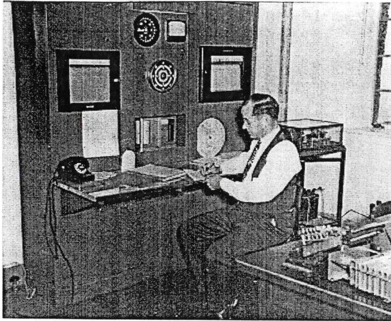
Figure 11. Observer logging a surface observation at a Weather Bureau Airport Station (WBAS) (circa 1935). Note modified version of the triple-register at far end of observer's console.
