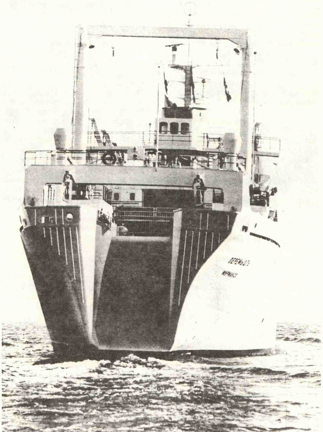
Photo 2. Fisheries training vessel Pelengator was launched in Denmark in 1968 for Soviet Pacific fishermen. This 102-meter long stern freezer trawler is used to train young students in the use of modern fishing gear.
