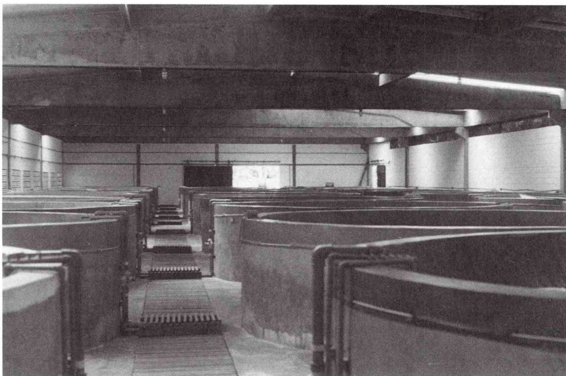
Photo 16.--Brazil. This hatchery has been modernized with a closed circulation saltwater and inverted photo period system. © Sergio Luiz de Siqueira Bueno, LPC/USP
