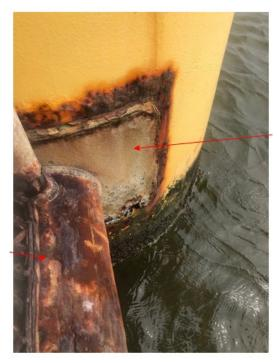
Figure 15. – Corrosion issues at the Calcasieu Pass SPIP boat landing doubler plates and support pipe beams
