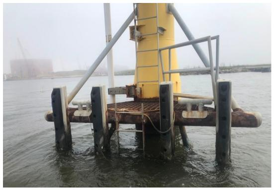
Figure 14. Corrosion issues on the Calcasieu Pass SPIP boat landing
