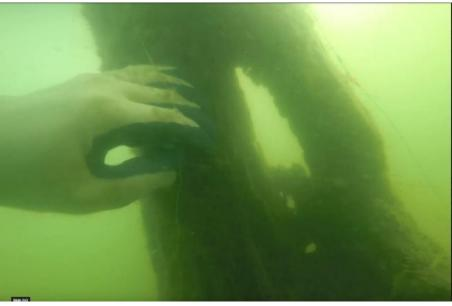
Figure 11. Dauphin Island Base platform damage found in an underwater survey of the station's timber piles
