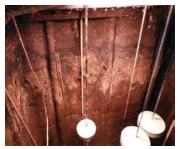
Figure 13. Ogdensburg, New York station sheet pile corrosion
