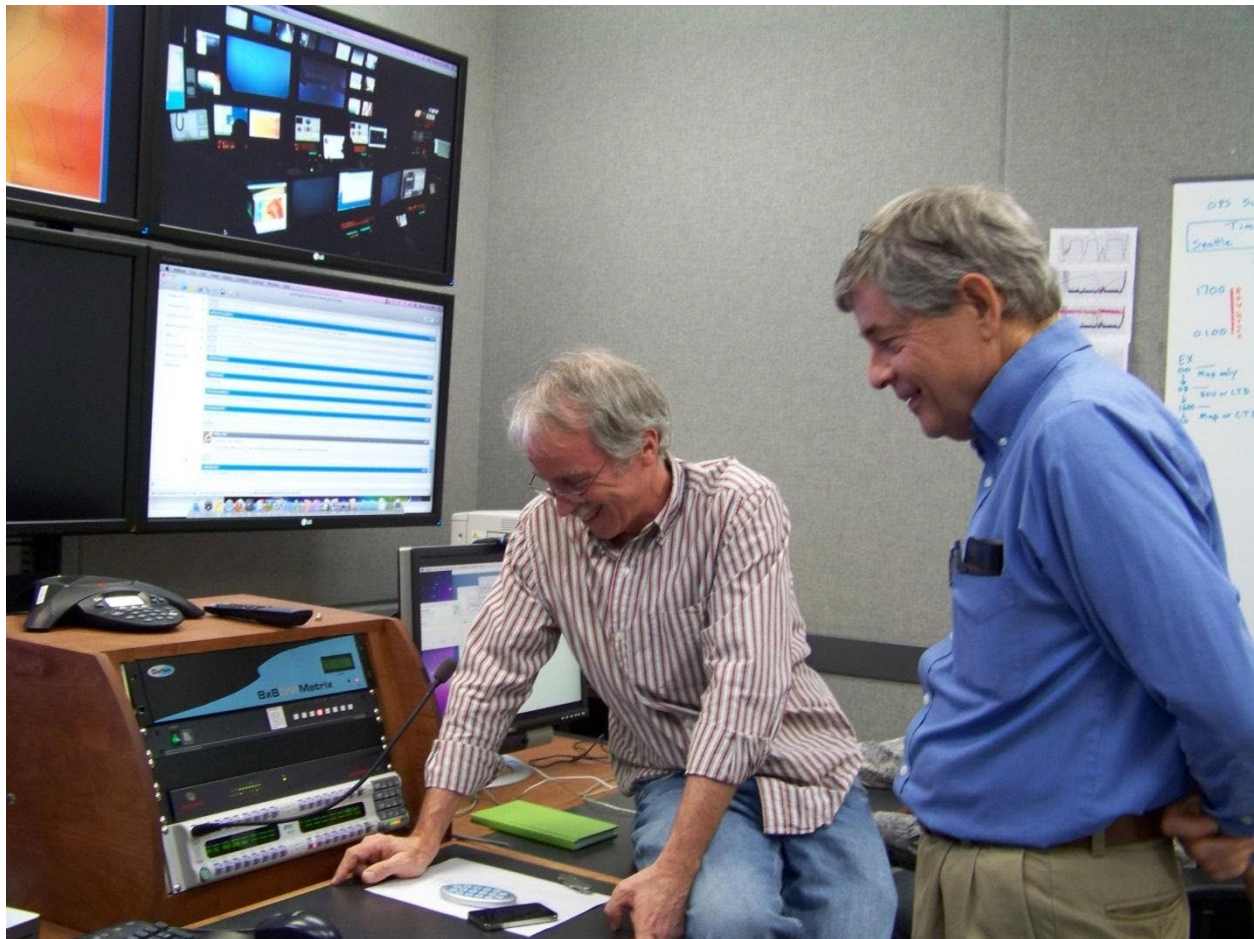
Figure 11. Voice communication between Okeanos Explorer and shoreside ECCs uses a VoIP-enabled RTS intercom system. The intercom system leverages the Okeanos Explorer's Internet connectivity to connect all of the ship-based and shore-based intercom units into a single system.
