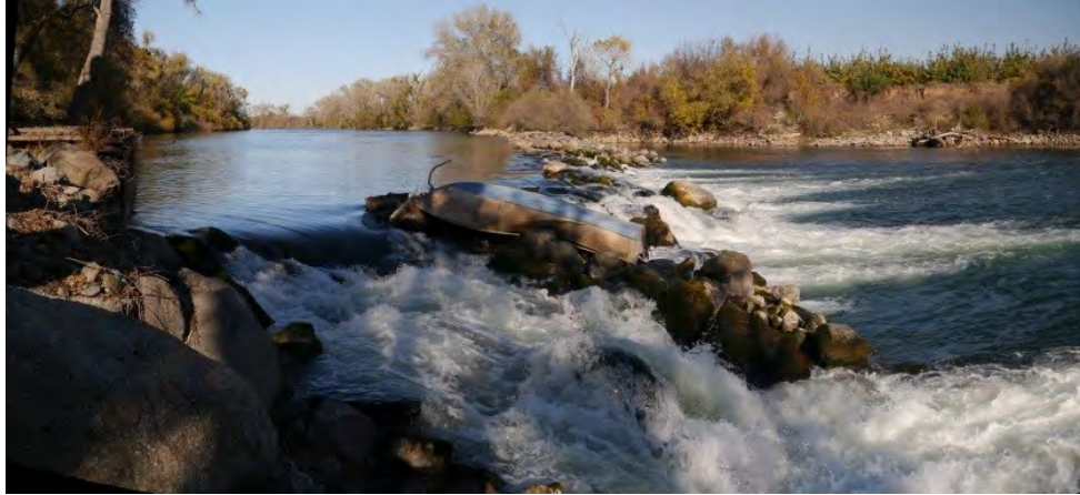
Figure 8. Photo of the Boulder Weir at Sunset Pumps.
