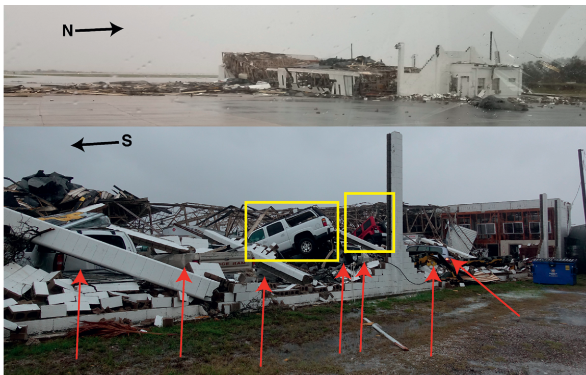
Fig. 7. Damage to buildings and cars (yellow boxes) near the DOW8 location at the Aransas County Airport (Wurman and Kosiba 2018).
