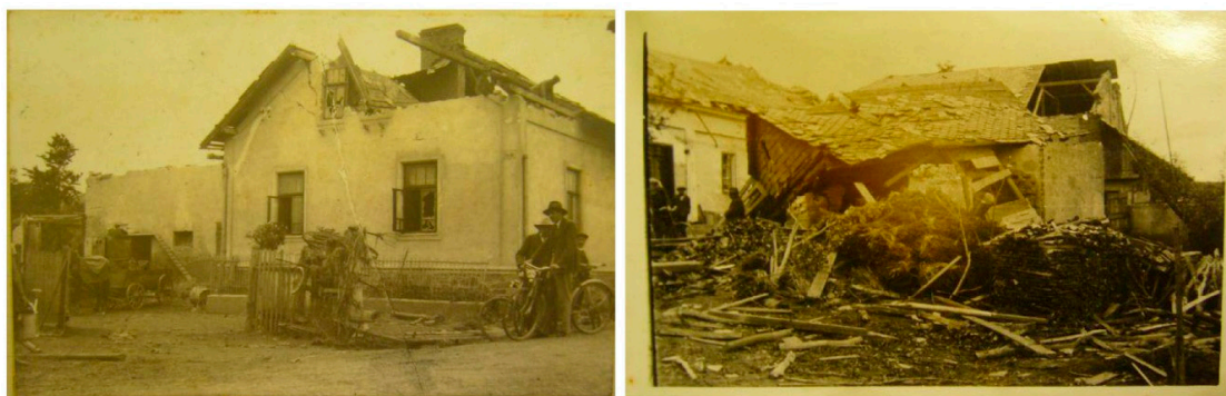
Figure 2. Buildings damaged during the F3 tornado in Milostovice on 21 June 1932 (source: [73]).
