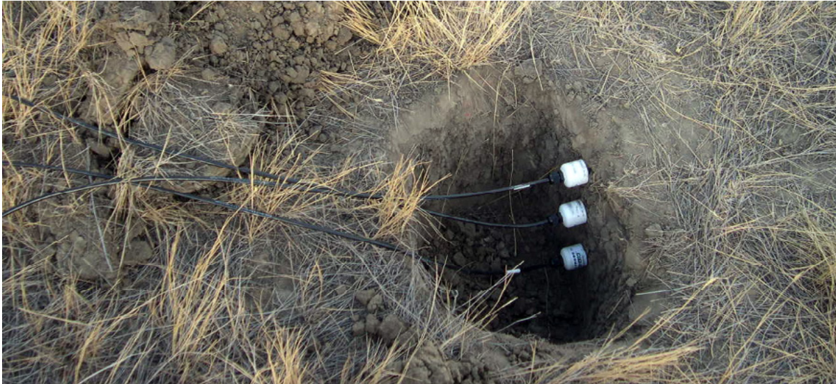
USCRN soil moisture station installation, Fort Peck Tribes Reservation, Montana. Credit: Tilden Meyers
