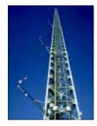
OAR - ETL - BAO **Boulder Atmospheric Observatory** The BAO is a 300m research tower measuring winds, temperature, and RH at 5 levels.
