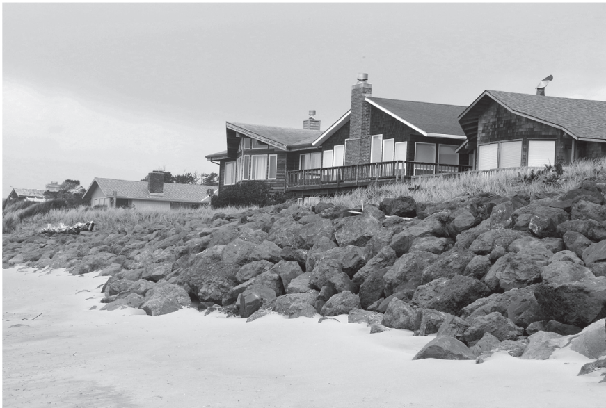
Fig. 2. Example of a shoreline protective structure. A rip-rap revetment in Neskowin, Oregon in April 2018. Photo by Steven J. Dundas.
