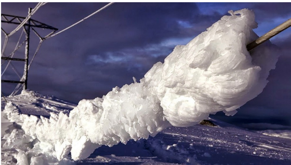
Fig. 1. Collapsed transmission line at Ålvikfjellet in January 2014. The ice loads were measured to 68 kg/m. Photo: Ole Gustav Berg, Statnett.
