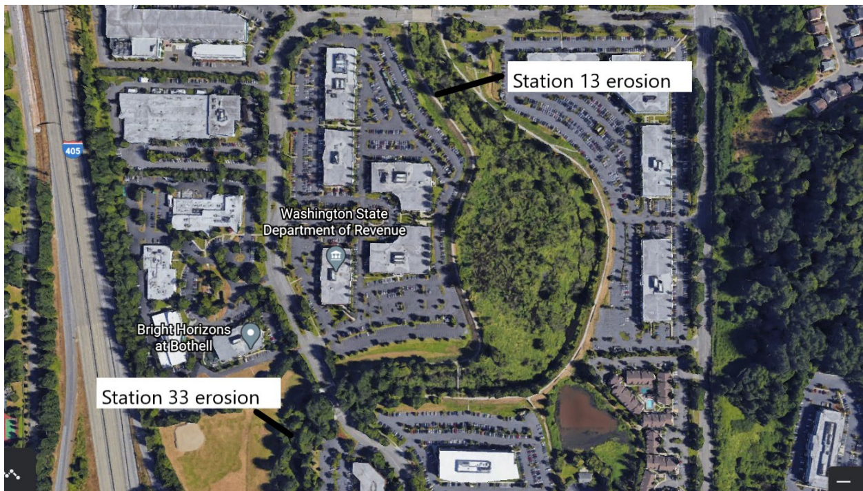
Figure 1. North Creek levee repair site showing locations of stream erosion (Station 13 and 33). Credit: Google Earth.
