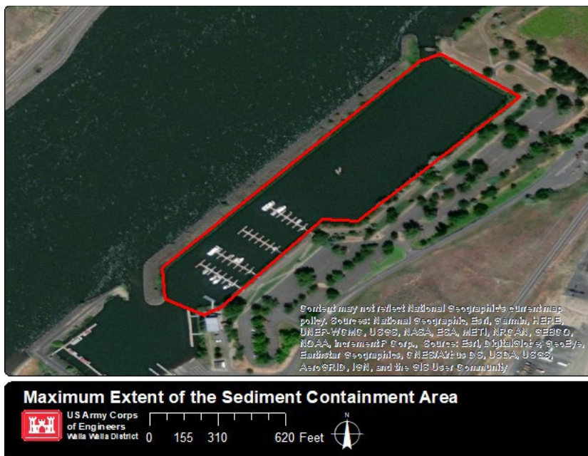
Figure 3. Outlined in red is the largest portion of the boat basin that would be isolated using sediment curtains.
