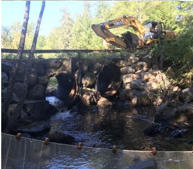
Figure 5.3.4. Jellison Meadow Brook crossing, before (left) and after (right), Mariaville, 2020. (photo credit: Ben Naumann, NRCS)
