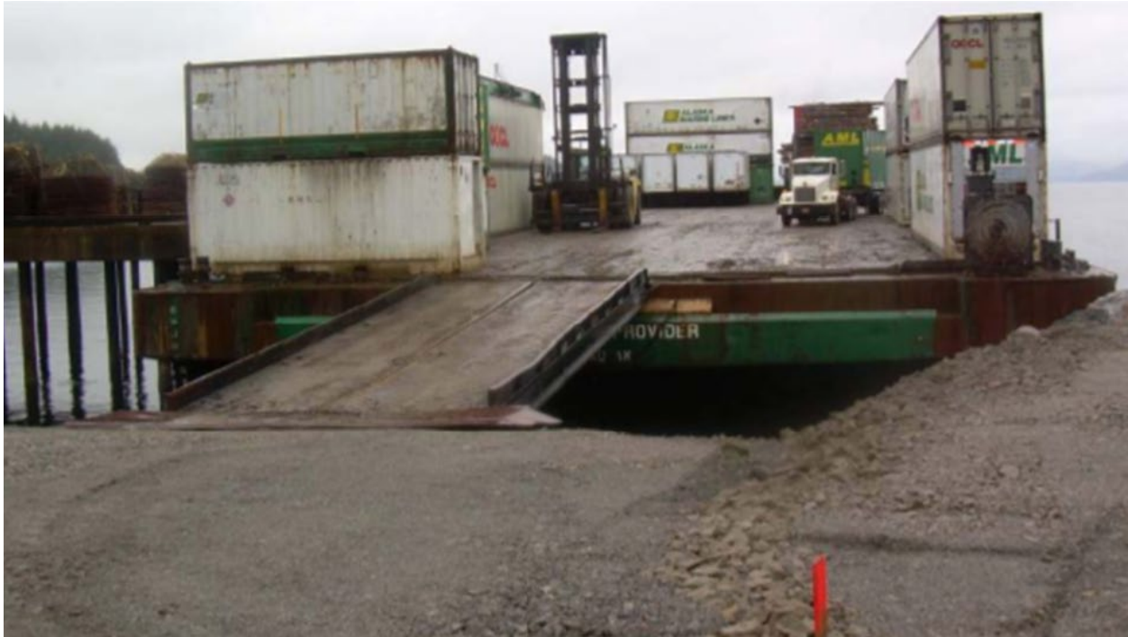
Figure 3. View south from the current gravel loading ramp.
