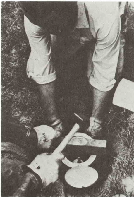
15 Driving the protective pipe into place.
