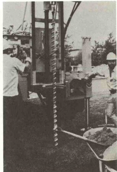
6 Drilling a hole for the sleeve.
