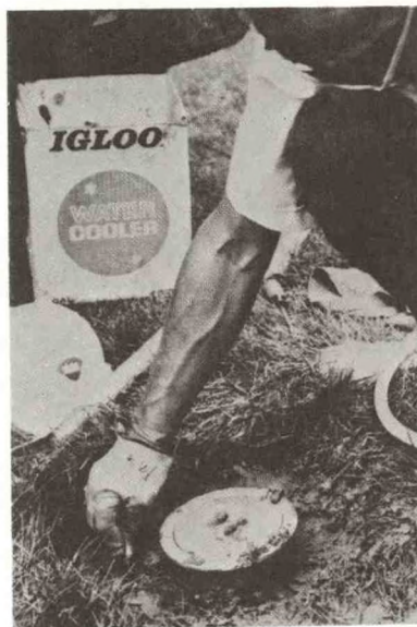
18 Working concrete around the protective pipe and logo flange.
