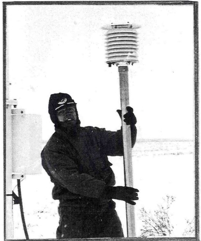
Figure 2. Terry Landsvork the Cooperative Program Manager installing a MMTS on the ASOS instrument array.
