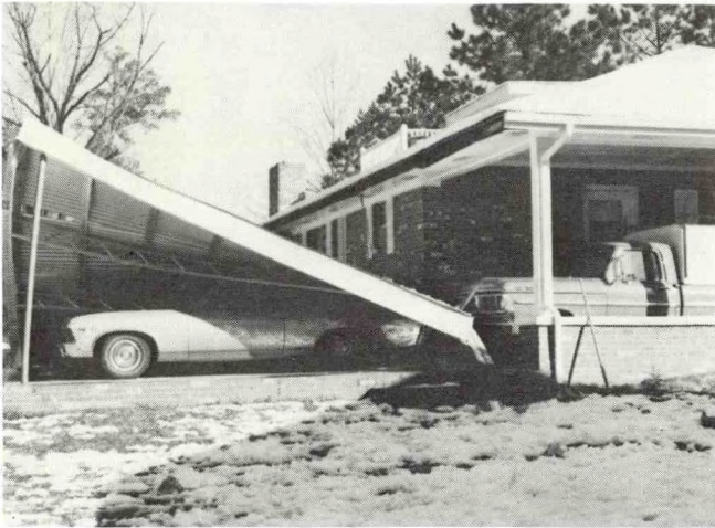
GREENVILLE, ALABAMA. Two prefabricated awnings that collapsed causing damage are shown. Photos Courtesy of Greenville Advocate .
