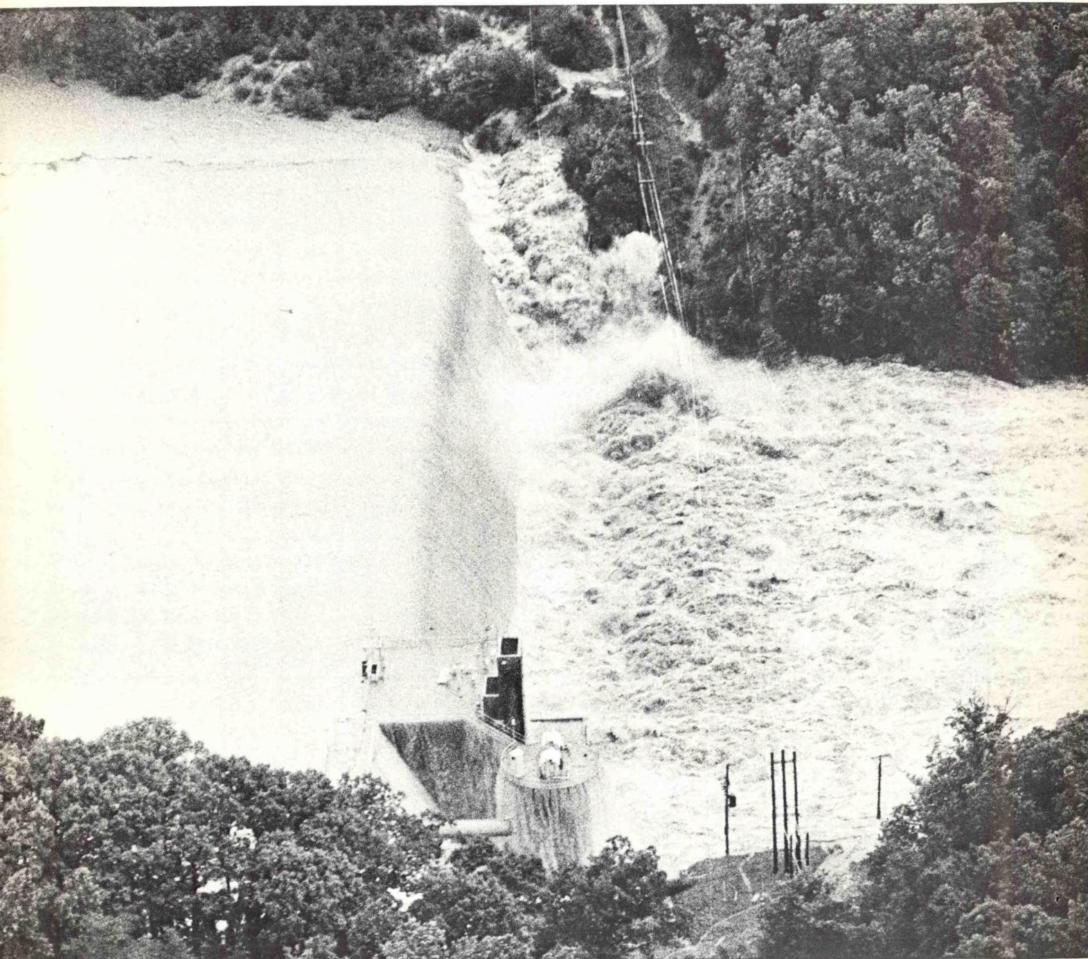
Flood waters caused by the rain from Tropical Storm Agnes boil around both ends of the 125 foot high dam at Occoquan, Virginia, southwest of Washington, D. C. At the time of the picture, water was topping the dam by 10 feet. (Wide World Photos)
