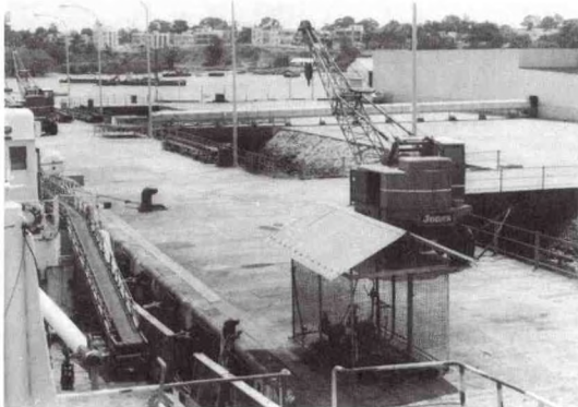
Photo 4.--View of KFI's dock area and conveyor belt system. A ship repair facility is visible to the left of the main freezing plant.
