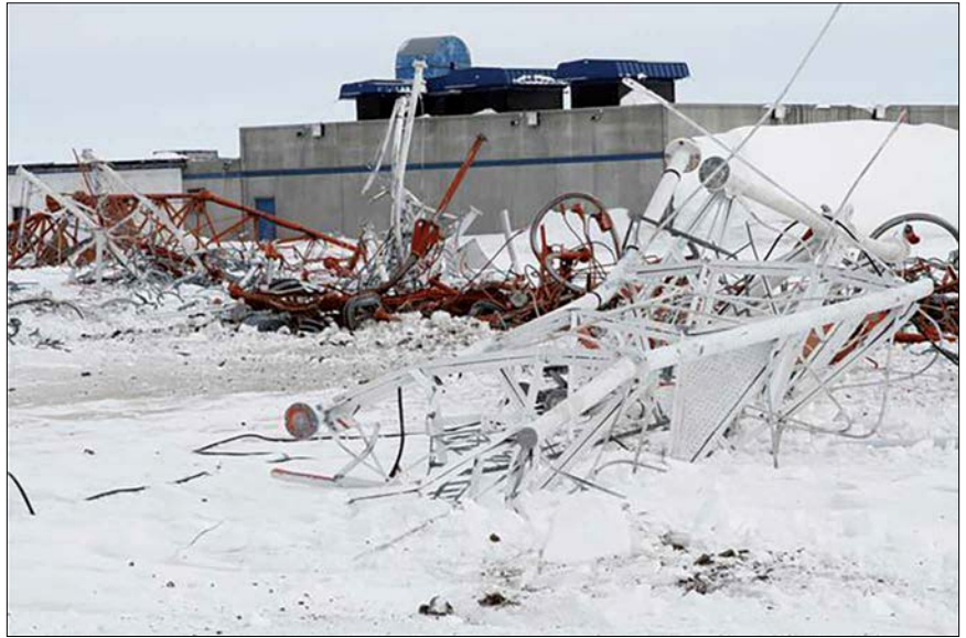
Alaska's tallest structure in Port Clarence, Alaska, a deteriorating Long-Range Aids to Navigation tower, was brought down more than 10 years ago. Additional aids to navigation are just one component needed for the United States to successfully expand its Arctic presence. Coast Guard photo by Jim Wells
