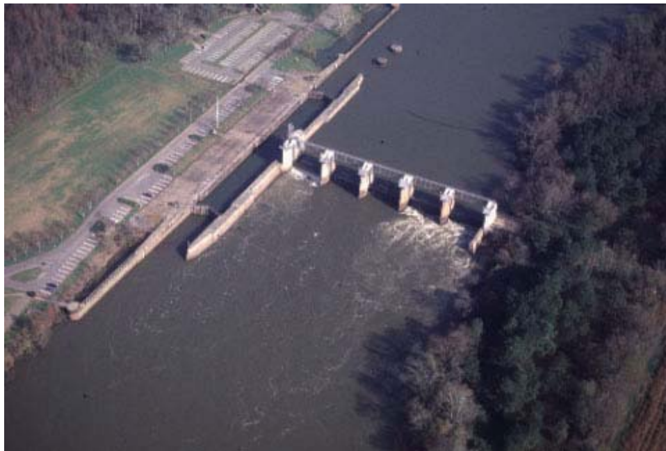
Figure 6. New Savannah Bluff Lock and Dam
