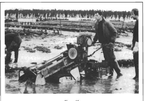
Figure 15 Motorized equipment for harvesting cultured clams in soft bottom and small-acreage leases.
