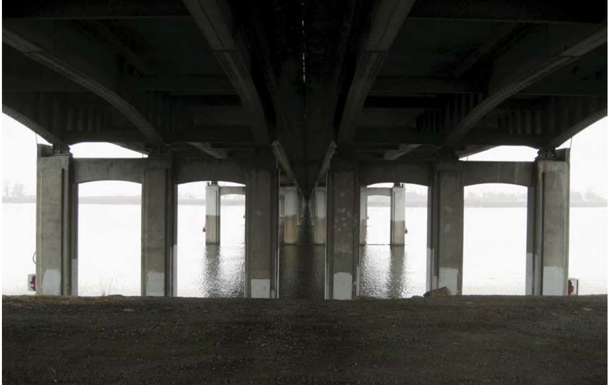
Figure 2: View of the underside of the bridge.
