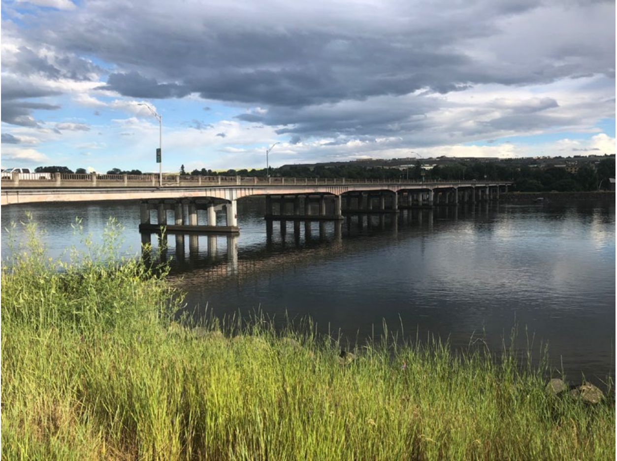
Figure 1: Side view of existing bridge.
