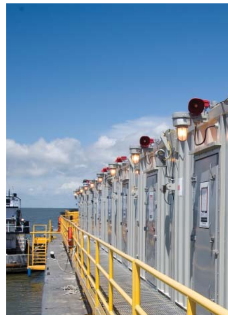
GRAND ISLE, La. – A tug is moored to a floating hotel (flotel) which houses approximately 80 contract workers for the Deepwater Horizon response. The flotel provides a galley, laundry facilities, television, rooms, and wireless internet. Photo courtesy of U.S. Coast Guard
