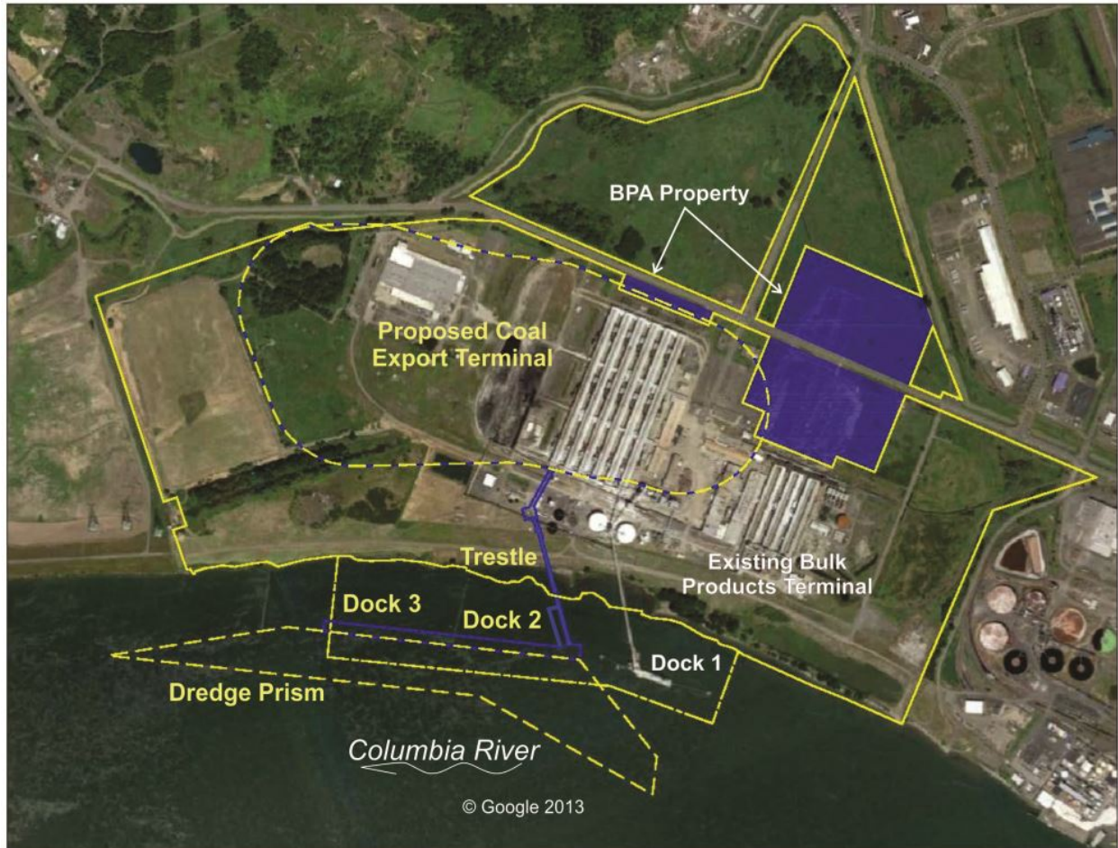
Figure 2. Project location within the MBT-Longview industrial area.
