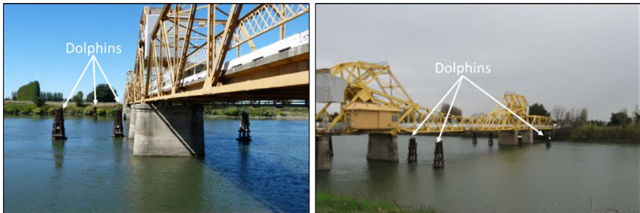
Figure 2. Existing dolphins at Paintersville Bridge (from Caltrans 2016).
