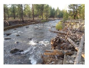
Figure 9. Constructed riffle on Whychus Creek, Oregon.
