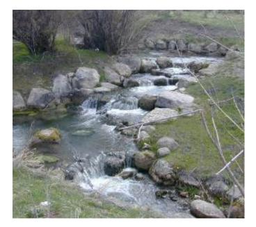
Figure 12. Constructed Step-Pool (photo courtesy of Rob Sampson).
