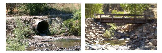
Figure 1. Original undersized culvert and subsequent bridge replacement.
