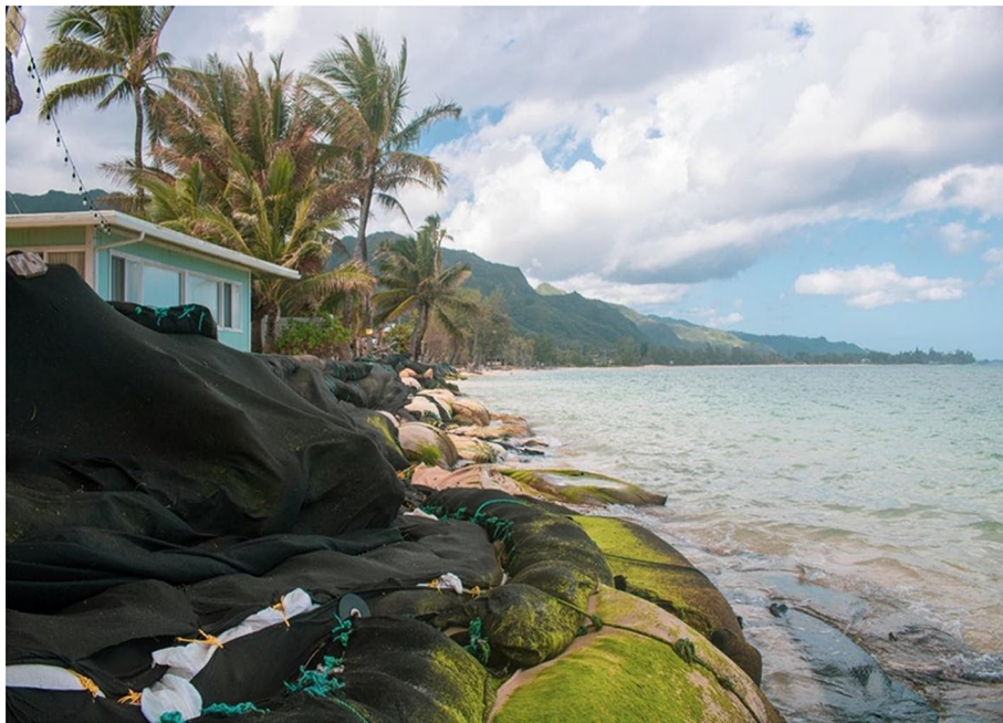
Figure 1. Hardening to protect backshore assets has resulted in widespread beach loss in Hawai'i. Photo of Ko'olauloa shoreline in March 2020 provided by contributing author Kammie-Dominique Tavares.
