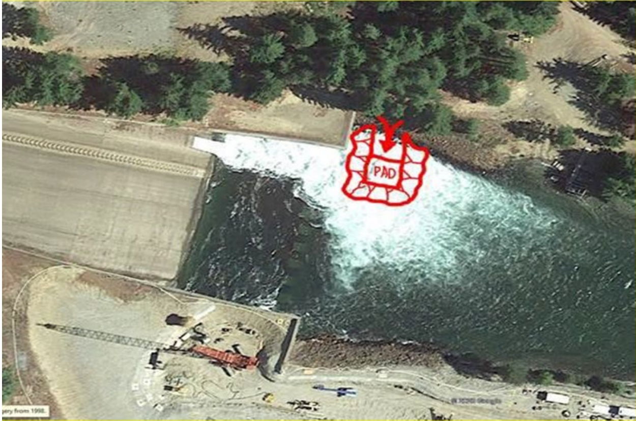
Figure 3. Temporary crane pad (Reclamation 2020, their Figure 13).
