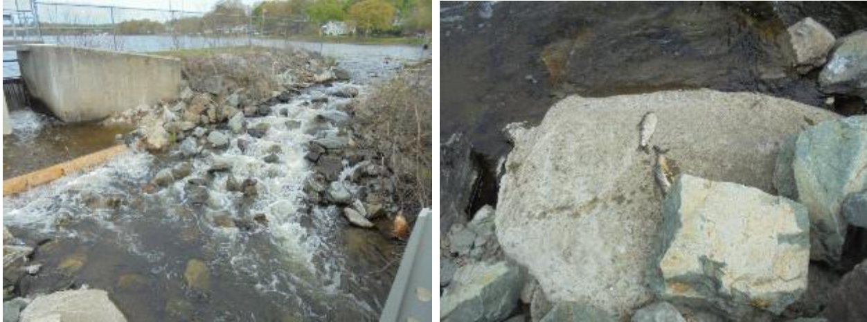
Photographs taken by Fuss & O'Neill at Scalley Dam on May 7, 2019.
