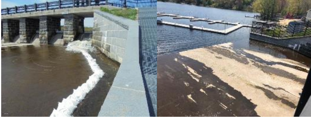
Figure 18. Mystic Lake Dam and Shallow Flow onto Spillway (right image) and Sandbags Used as a Temporary Solution to Promote Fish Passage (left image)
