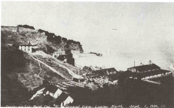
General view of the cove (looking north) during early construction of the Navy Coaling Station, Sept. 1, 1906 (courtesy Navy Dept., National Archives).
