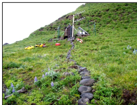
Figure 12. Pressure sensor tide gauge and tubing
